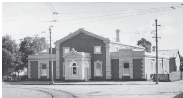
Fig. 4-5 Mitcham Institute, c.1950. The West Wing (seen on the left) and the Mitcham Boys' Club and Gymnasium (at the rear) were both built in 1900 whilst Reverend A.W. Clampett was President of the Mitcham Institute Assn. The Boys' Club was demolished in 1972 and the Mitcham Village Art & Crafts Centre now occupies the site. (MLHC, Arnott-Rogers Collection)
