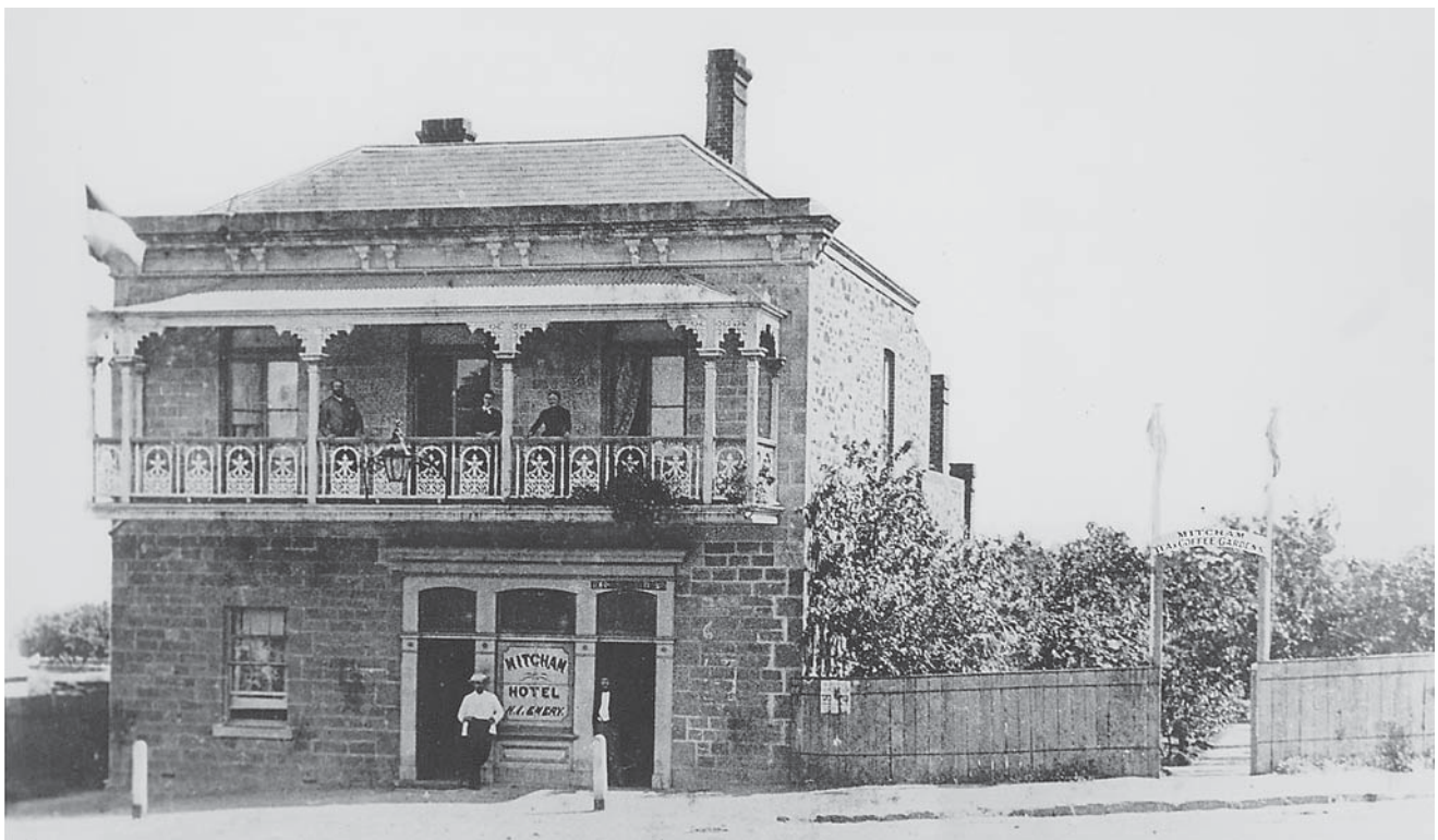
Fig. 3-3 The Mitcham Hotel, c.1885. Henry Taylor's former single-storey Brownhill Creek Inn was converted to two storeys in 1879 by John Wark. The architect was James Cunningham. On the right is the entrance to the Mitcham Tea and Coffee Garden. (MLHC)
