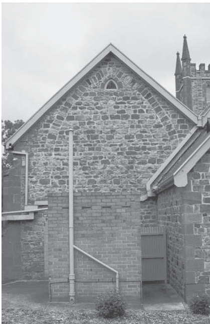
Fig. 14-5 The toilet block built in 1958. Note the 'blind arch' in the eastern wall of the south nave. (Ben Oborn, 2002)
