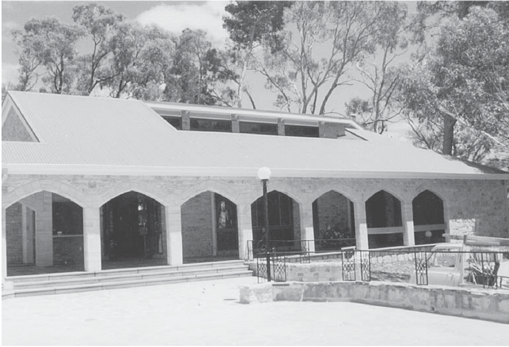
Fig. 14-14 Final clean-up on 29th November 1980 in readiness for the dedication by Archbishop Rayner the next day. (MPA)
