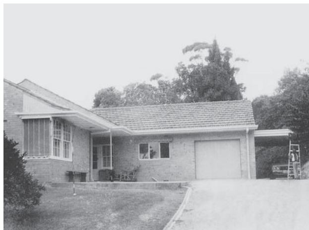
Fig. 14-6 The Rectory as it appeared in 1977 prior to the garage being converted to a separate family-cum-meeting room. In 1986 the walls between that room and the kitchen and back porch were removed to make a large kitchen/dining/family room area under the main roof. (Ben Oborn)
