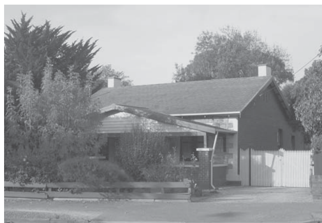
Fig. 13-10 St Wilfrid's Parish House, 2 Belair Road, Torrens Park, was purchased in 1961 for use as a future curatage or rectory. For twelve years it was leased to private tenants before being sold in 1974. (Pamela Oborn, 2002)
