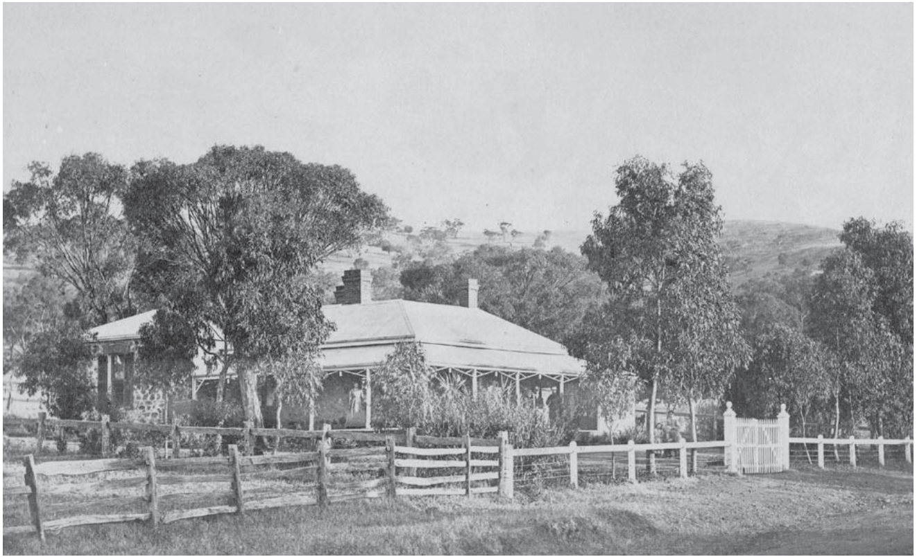
Fig. 14-1 The Parsonage c.1869. The entrance gates built about this period remained a feature of the property. (MPA)
